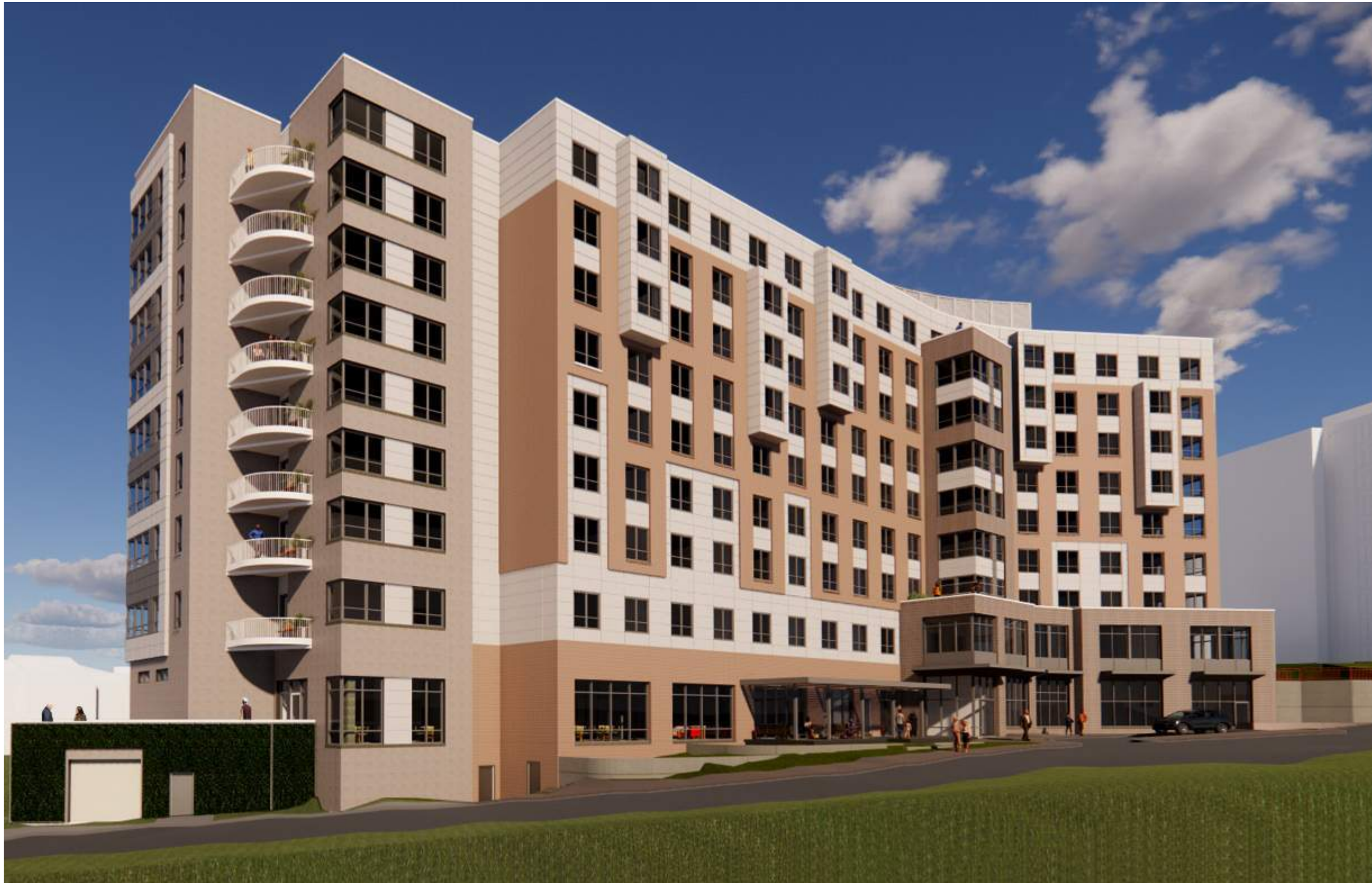
View From Adjacent Development (South West)
