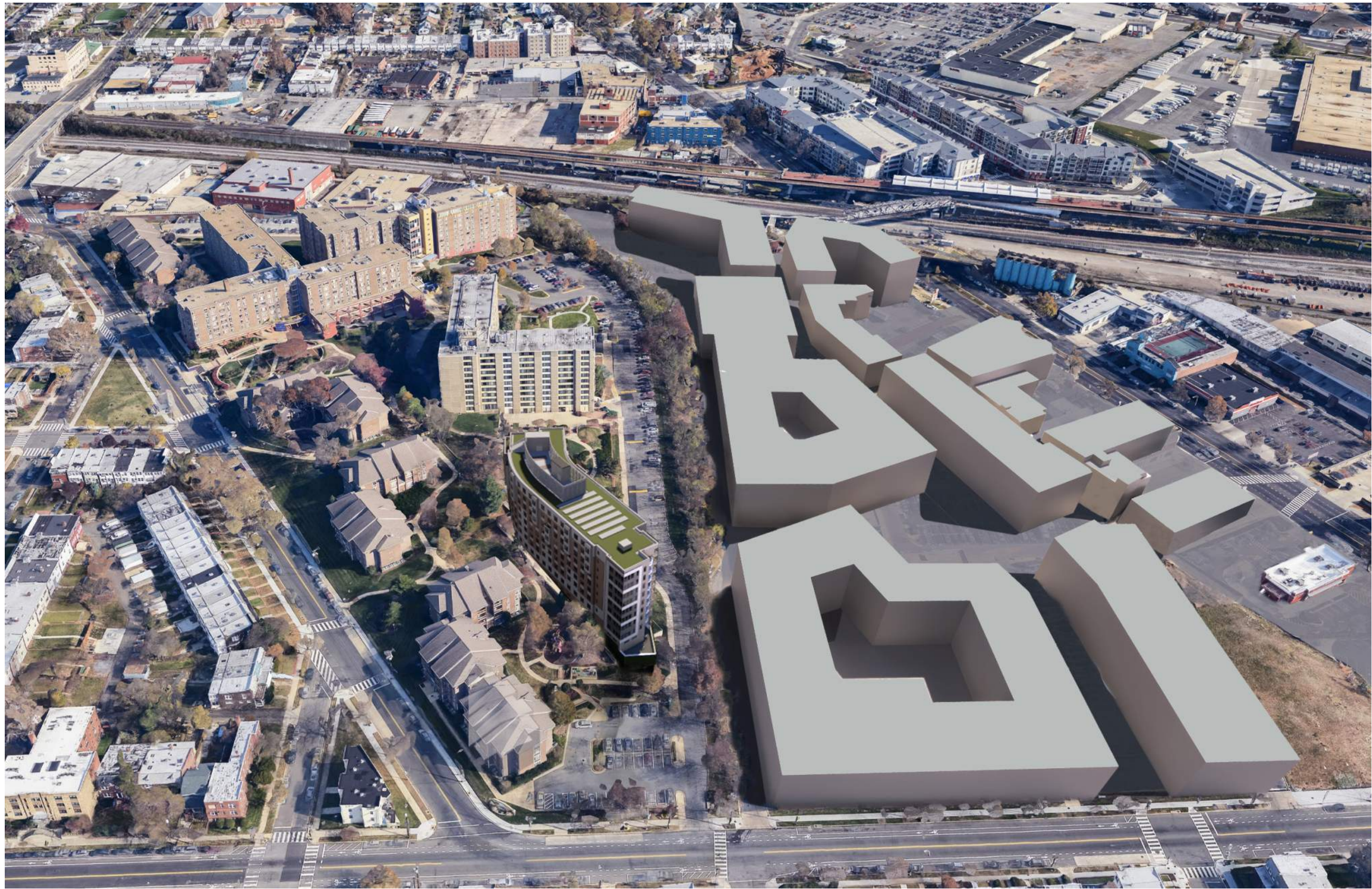
View From the West
