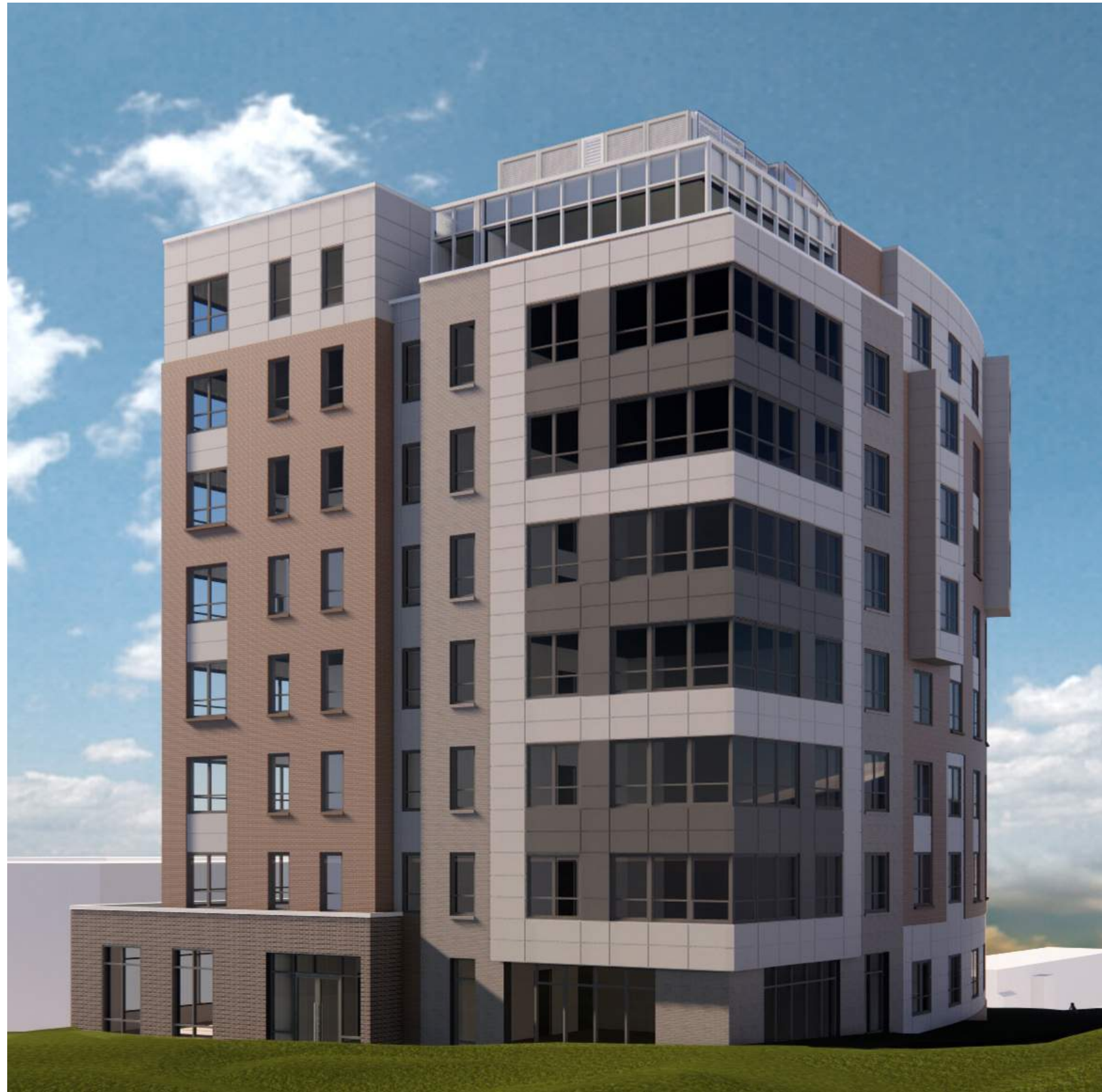
View From Edgewood Campus Interior (North East)
